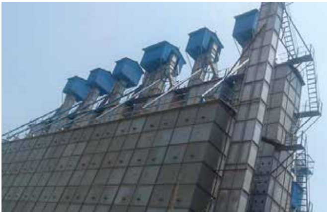
A project engaged in processing of different types of high quality rice financed by BASIC Bank Ltd, Khulna Branch
